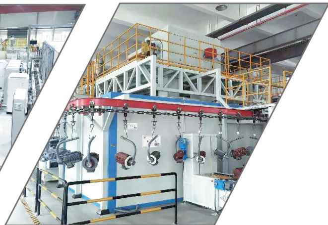
悬挂链电机喷漆线
