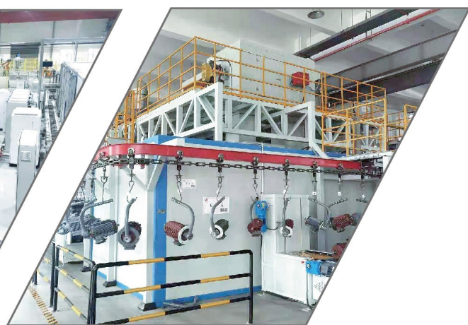
悬挂链电机喷漆线
